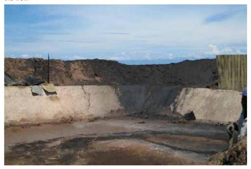
Photo 6: the damaged flare pit following the Kingfisher-1 well text, showing damaged steel sheets
