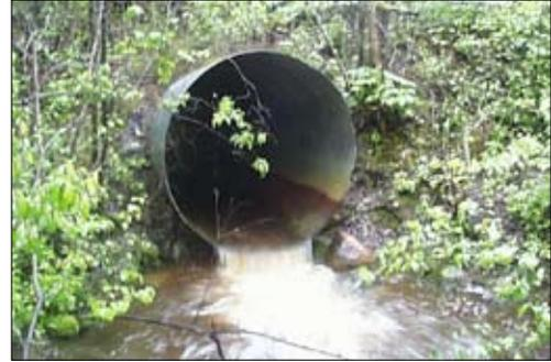
Improperly installed culverts can make it impossible for fish to move upstream.
